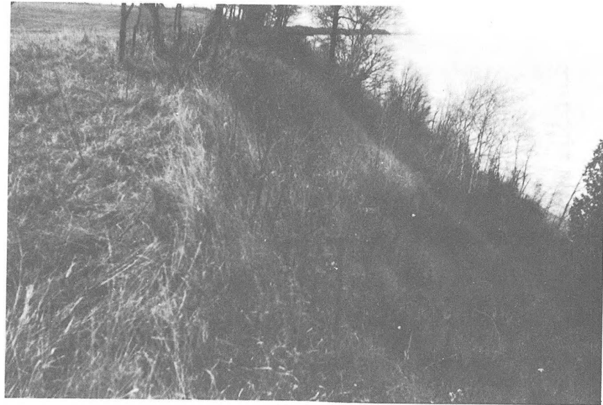
Figure 6. Lake Michigan bank erosion caused by seepage through sand and gravel layers in the glacial till (left). Dewatering, bank reshaping, and seeding to prevent erosion by runoff has stabilized bank recession (above). (Courtesy of Soil Conservation Service.)
