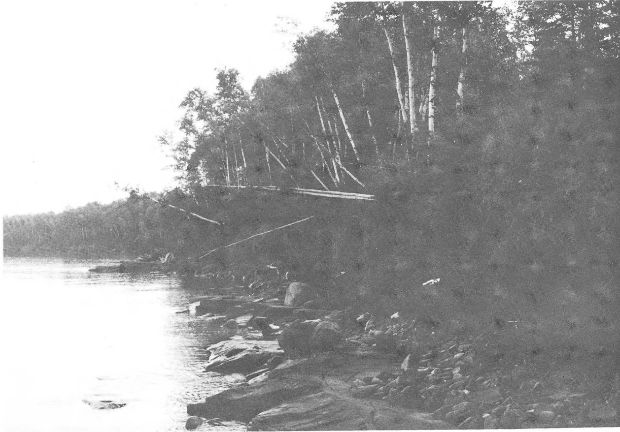
Figure 5. Wave scouring causes undercutting and bank recession with loss of vegetation.
