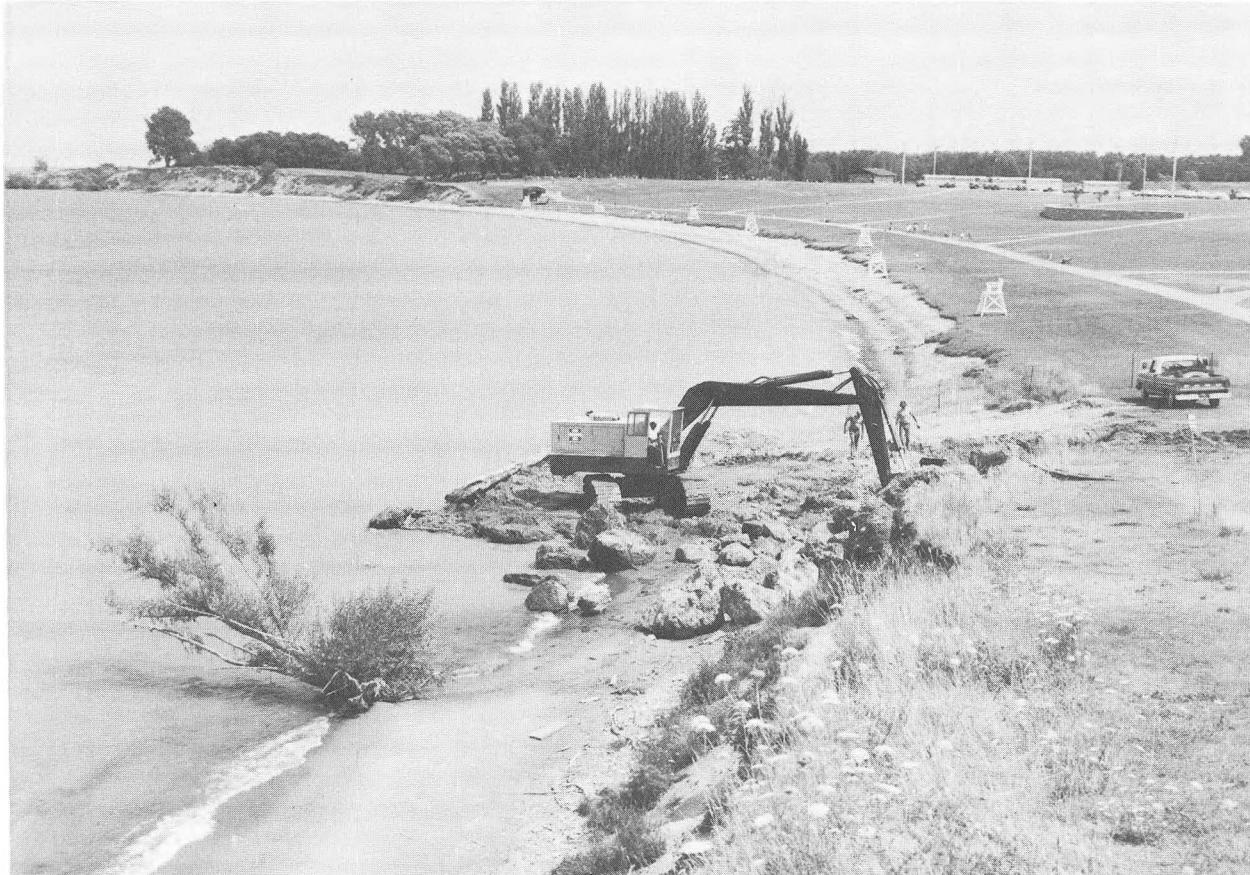
Figure 10. Landscaped beach area and parking lot developed by reforming a high eroding sandbank.
