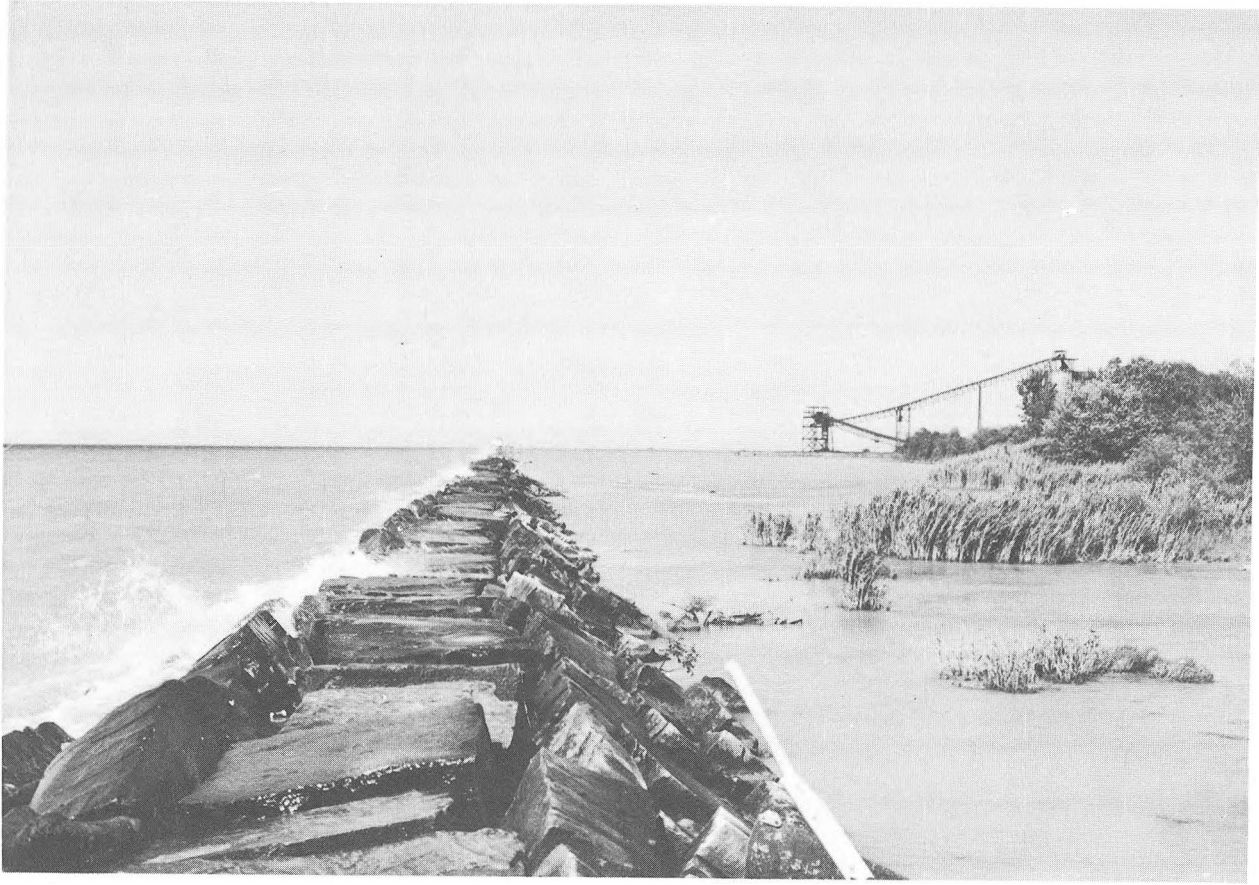
Figure 9. Protective structure creating pool favorable for growth of reed.
